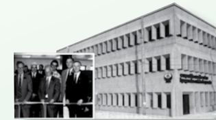
June 3rd 3rd floor added 950 Main St. 1981
